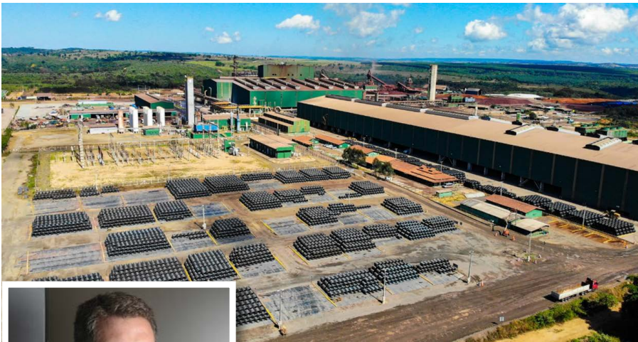
Fig 4. AVB Industrial Plant
